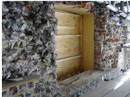
The Rose window above the sacristy entrance is being completely replaced
